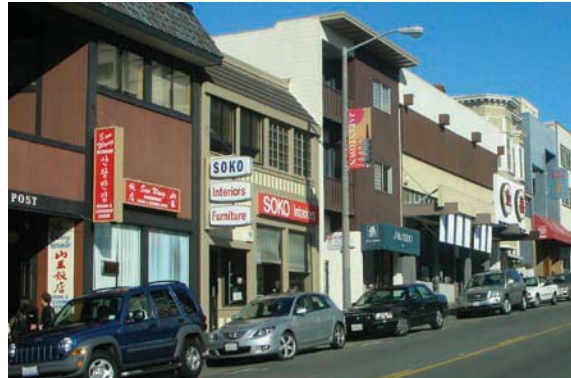
The block of Post Street between Laguna and Webster streets and Buchanan Mall marks the heart of the commercial district.
