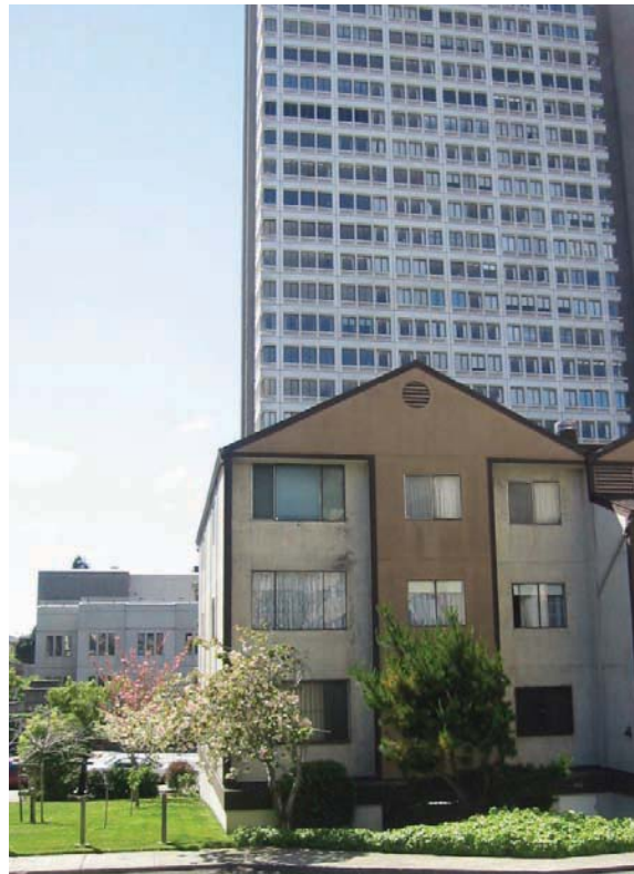
The Nihonmachi Terrace apartment complex (three-story townhouses in foreground) abuts the northside of Post Street and has a range of heights. The Sequoias residential tower is pictured in the background.
