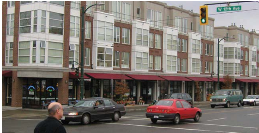
Material changes, bay windows, awnings, and individual store-fronts break up the mass of this building.
