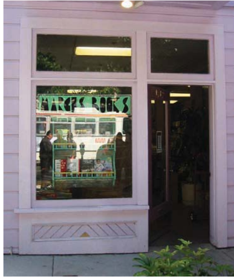
Marcus Books on Fillmore Street is on the first floor of mixed-use Victorian that was saved and relocated from Post Street during urban renewal.
